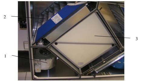
Fig. 2. Ventilation unit: 1 – fan; 2 – filter; 3 – heat exchanger for recuperation
