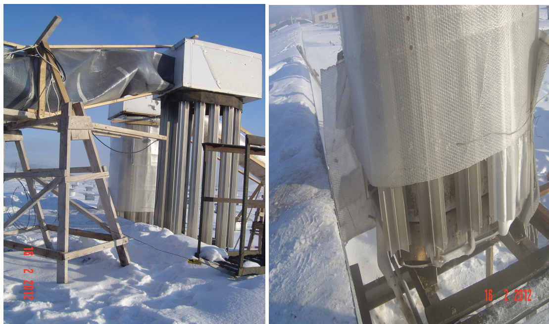
Fig.3. Heat pump evaporators during the experimental investigation. In order to see the heat transfer plates, the outside cover is opened (left side photo). At the bottom of the right side photo between two evaporator colons the location of the temperature sensor is seen
