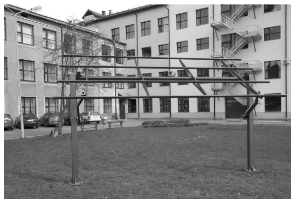
Fig. 5. Frame of alternative energy charging station
