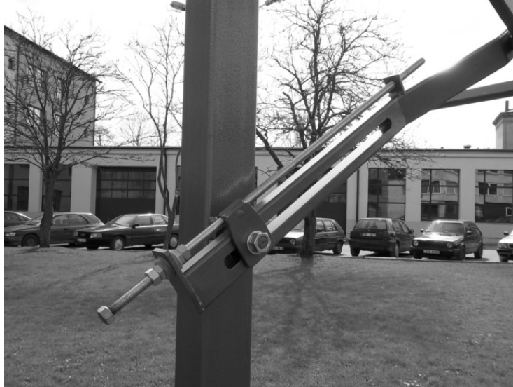
Fig. 6. Angle adjustment mechanism of the solar station
